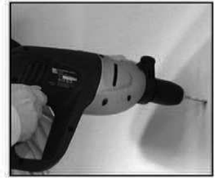
3. Remove the backplate and drill a 7mm hole.
