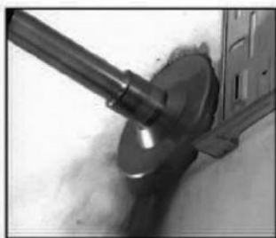
10. Drill the hole at a slight downwards angle. When you feel the pilot drill exit the outside wall stop.
