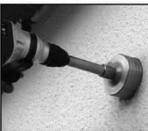
11. Finish the hole from the outside to keep it clean.
