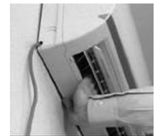
15. Lock the bottom of the unit onto the base of the backplate.
