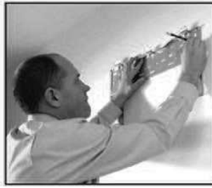
2. Mark the right hand backplate screw position.
