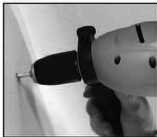
7. Drill the rest of the holes and insert the wall plugs.
