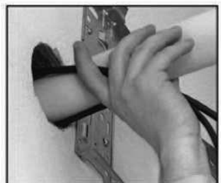
12. Feed the cord and drain hose carefully through the wall.
