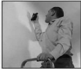
1. Check the area for any hidden wires or pipes.
