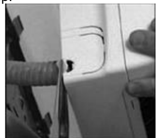
13. Undo the power lead and break out the plastic tab.
