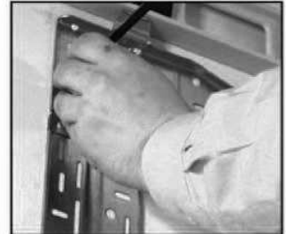
6. Check to ensure level, then mark the other holes and swing the backplate away.
